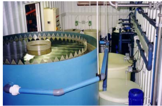
Containerised Packaged plant to treat raw river, dam or well water for domestic use in China.
